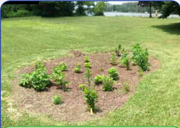
Figure 16: Rain gardens slow and filter pollutants such as bacteria, nutrients, and metals from stormwater runoff, while also beautifying the landscape. Rain gardens are often used in conjunction with rain barrels, which store rain until you need it. This demonstration rain garden is located at Old Trinity Church in Church Creek, Maryland.
