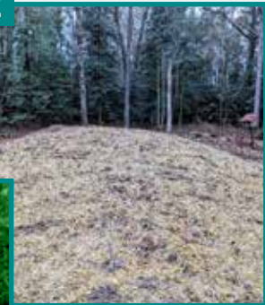
Pictured below: A septic mound that has been recently seeded with a septic safe wildflower mix.
