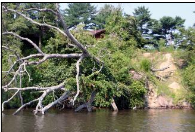
Erosion on the bank of the Nanticoke River in Delaware. July 2008. Photo by Don Allen.
